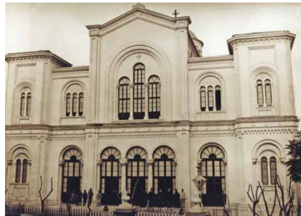
The Church of St Catherine, the largest in Smyrna, designed by the Smyranean architect Xenophon Latris Enosis Smyrnaion
